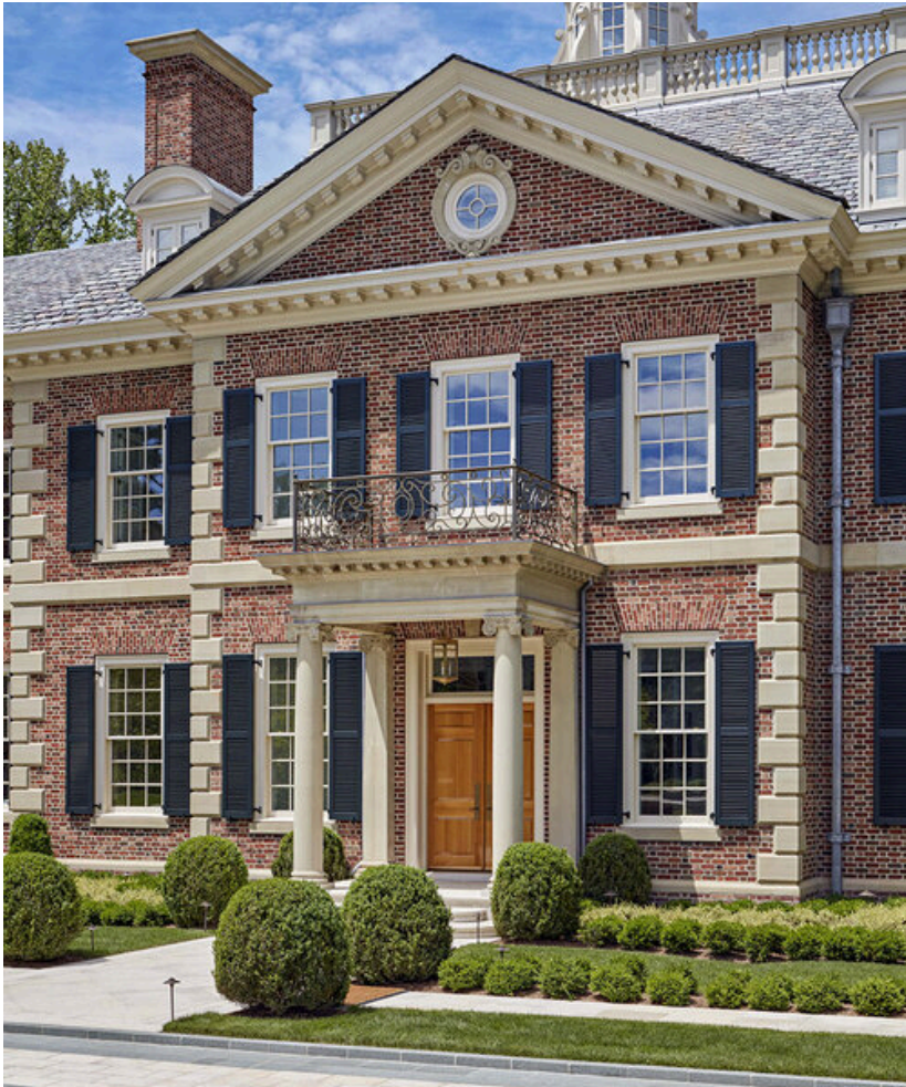
- The corner masonry
